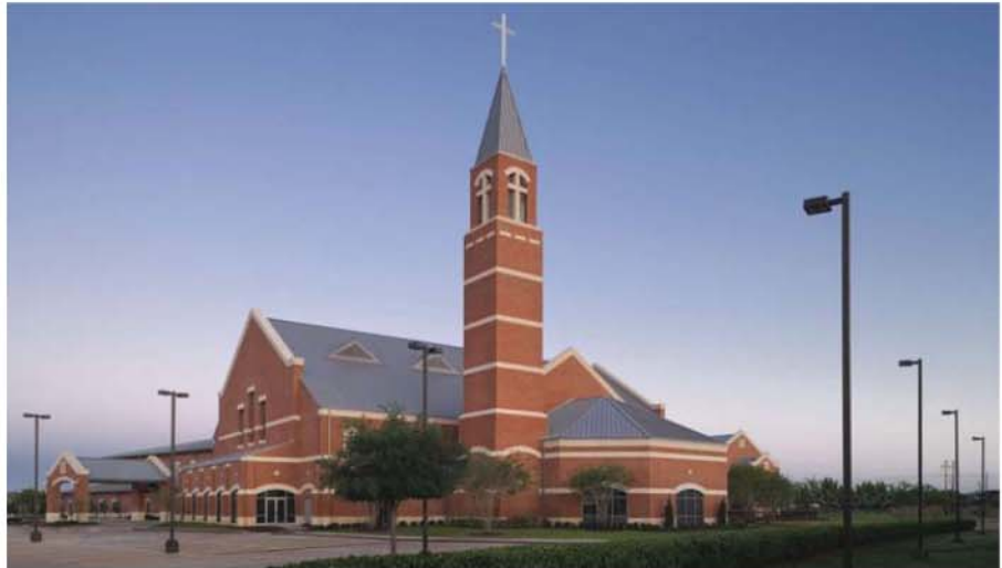
The recently completed First Colony Church of Christ in Sugar Land. The worship center was built by Fretz Construction and designed by Turner Partners Architecture. Photo: Aker/Zvonkovic Photography.
